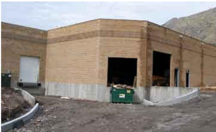
South of the existing building, the external part of the shipping and receiving addition is near completion. Adding a third dock, changing the locations of the docks and driveway, and adding a hydraulic lift on one dock will make access to shipping and receiving easier, especially for long trailers.
