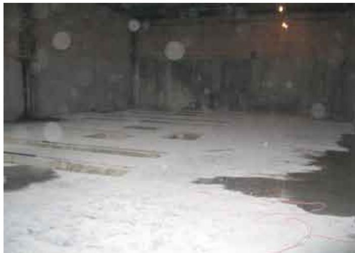
Dust in the air, seen as spots on this photo, will be eliminated by the new state-of-the-art down draft system to be installed in the paint booths. This area will house three booths for finish paint and a mixing room as well. The expansion of our paint area will improve the ability to manage multiple colors simultaneously.
